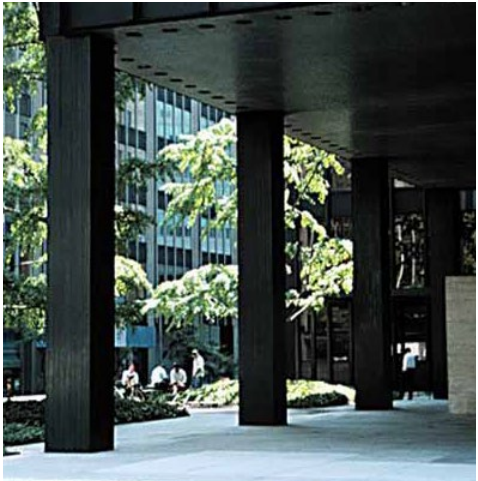
6. METAL CLADDED COLUMNS
