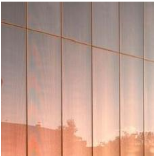
4. DGU WITH MESH INTERLAYER
