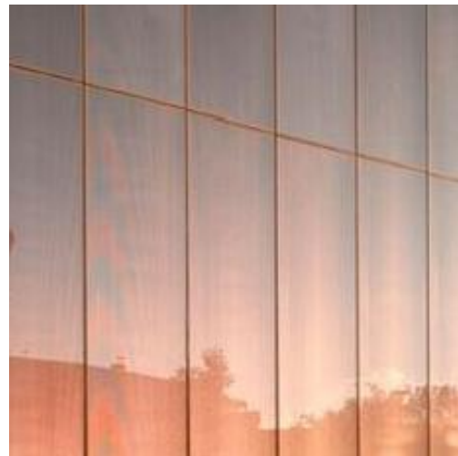
4. DGU WITH MESH INTERLAYER
