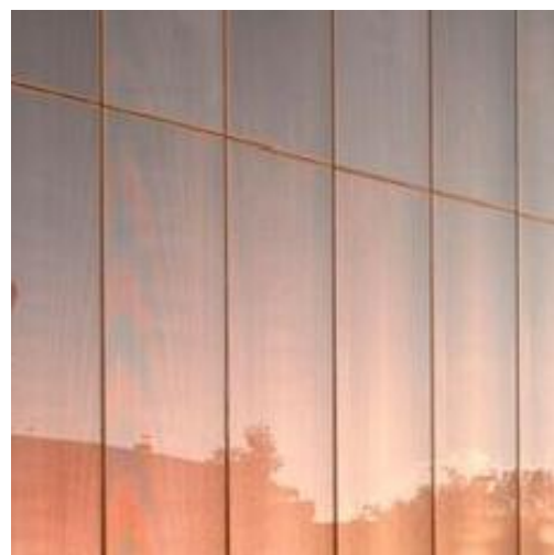
4. DGU WITH MESH INTERLAYER
